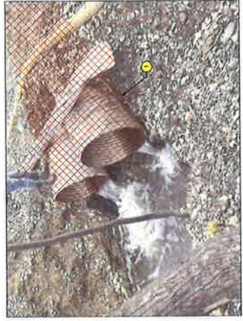
1 CULVERT OUTLET DEMOLITION NOT TO SCALE
