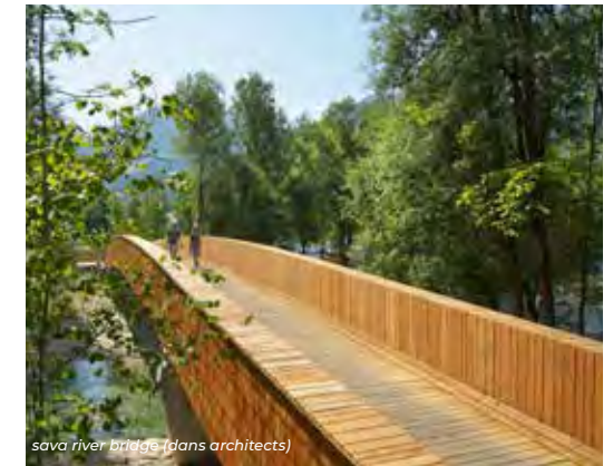
sava river bridge (dans architects)
