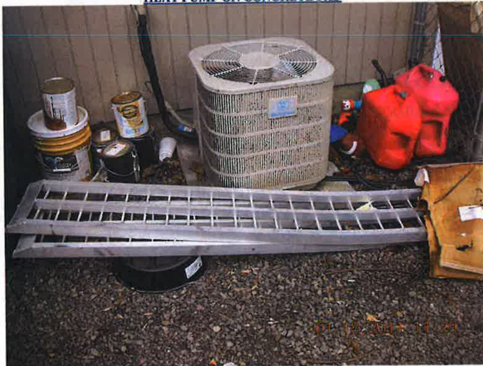
HEAT PUMP ON CONCRETE PAD
