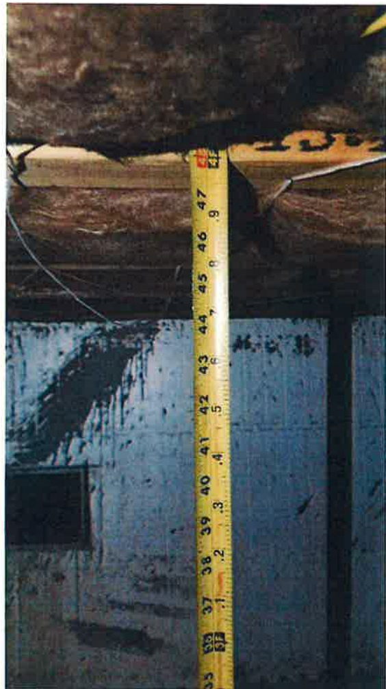
2018-02-14: CRAWLSPACE HEIGHT MEASUREMENT (NEAR NORTHEAST CORNER OF CRAWLSPACE)
