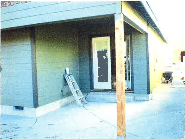
West side and back, vents visible ( Sept. 9, 2015 )
