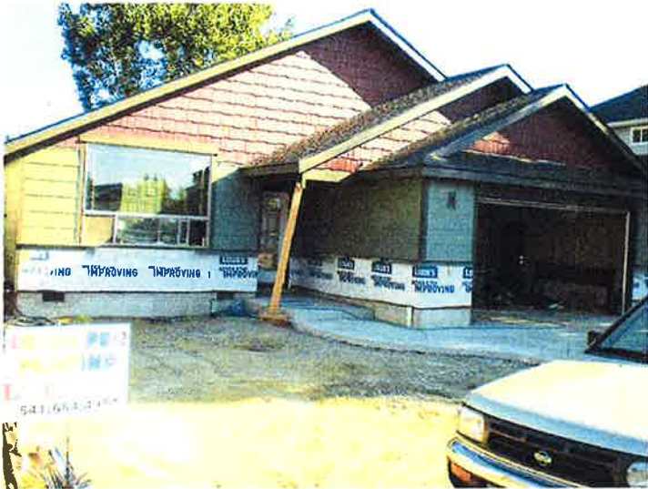
Front of house, vents visible ( Sept. 9, 2015 )
