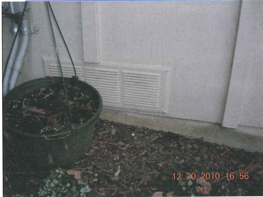
TYPICAL FOUNDATION VENT WITH LOUVERED COVER
