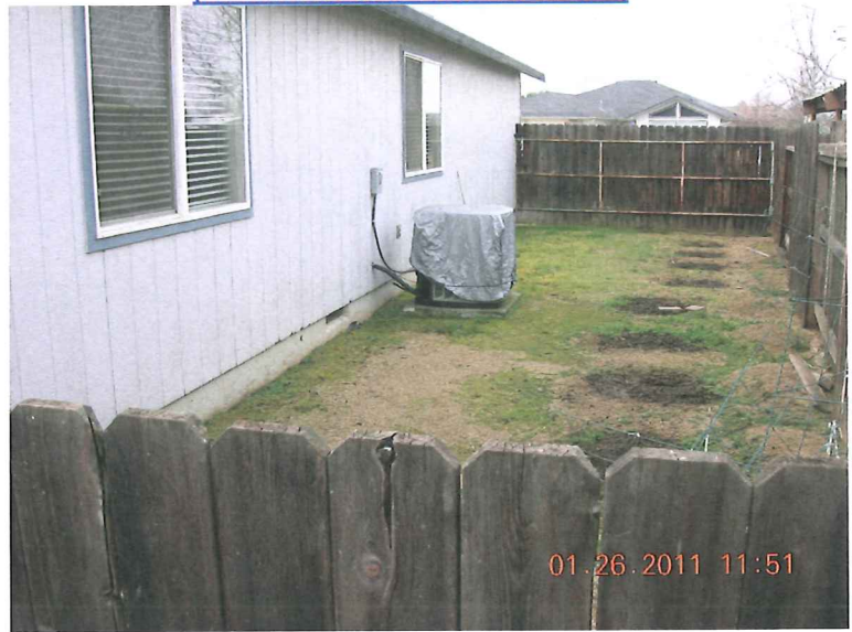
HEAT PUMP ON CONCRETE PAD (AT NORTHERLY FACE OF HOME)
