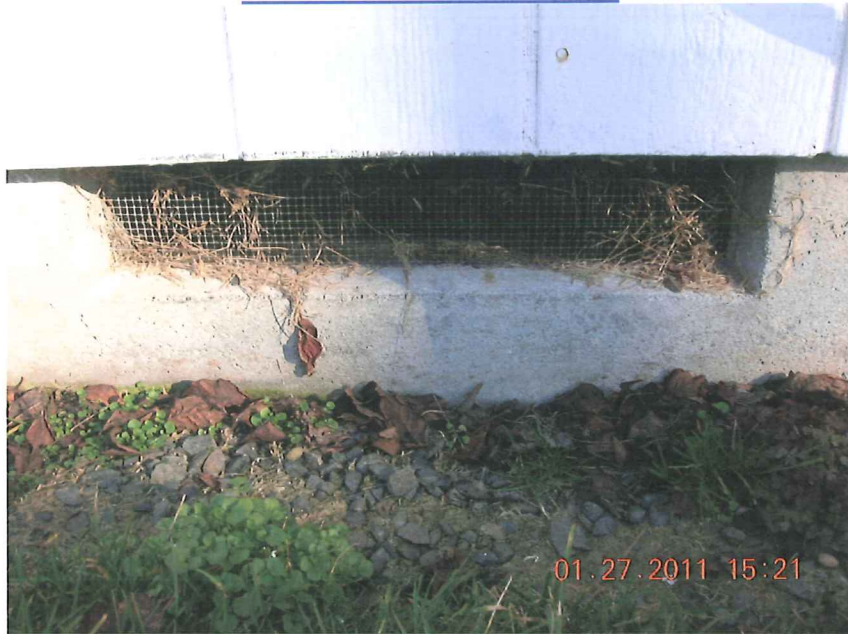
TYPICAL FOUNDATION VENT
