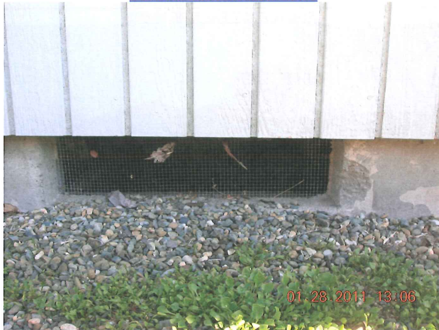
TYPICAL FOUNDATION VENT
