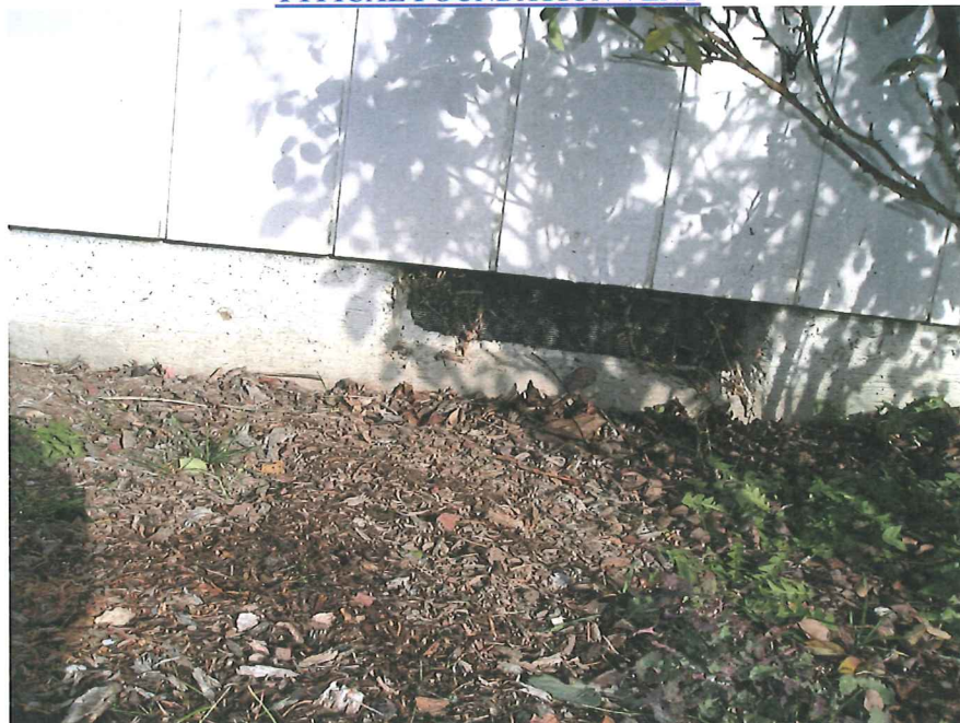
TYPICAL FOUNDATION VENT
