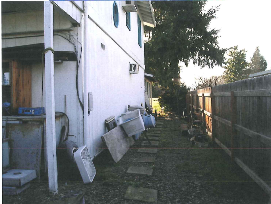
WEST FACE OF HOME (LOOKING SOUTHERLY)
