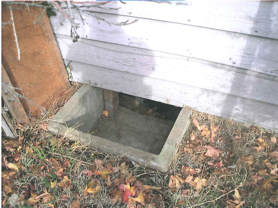
CRAWL SPACE ACCESS
