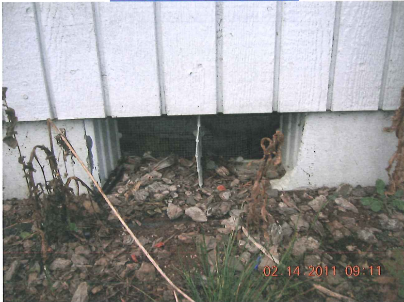
TYPICAL FOUNDATION VENT
