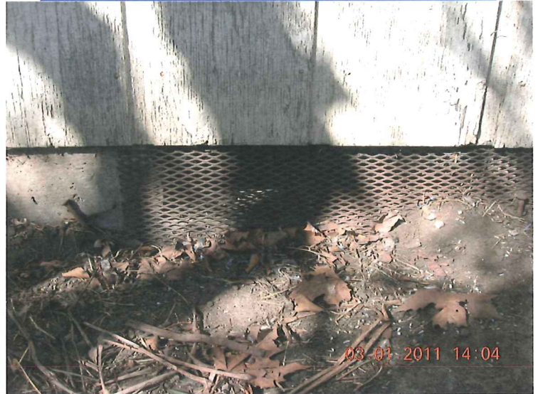
FOUNDATION VENT WITH METAL COVERING (3)
