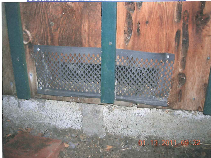
FOUNDATION VENT WITH METAL COVERING (2)
