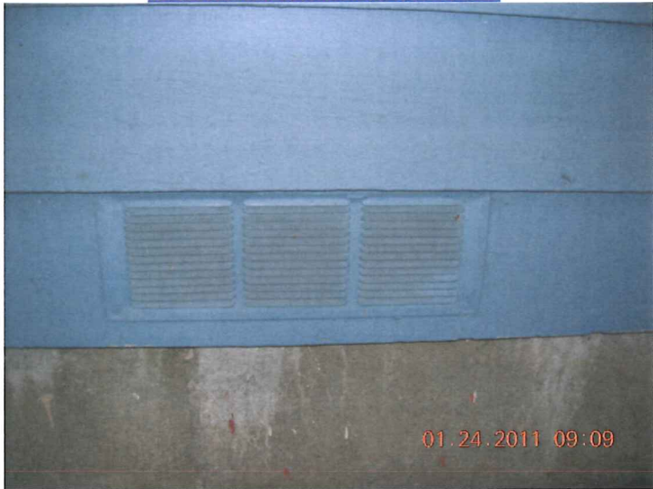
TYPICAL FOUNDATION VENT
