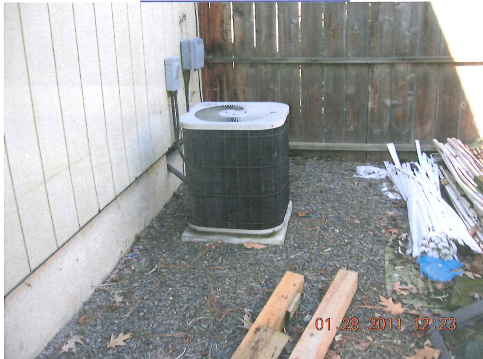
HEAT PUMP ON CONCRETE PAD
