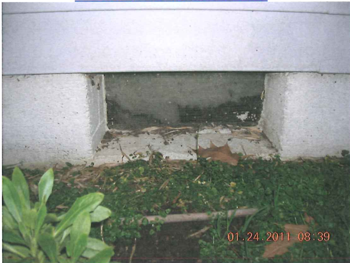
TYPICAL FOUNDATION VENT
