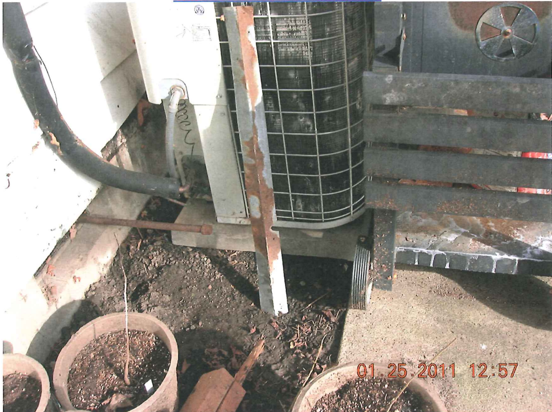
HEAT PUMP ON CONCRETE PAD
