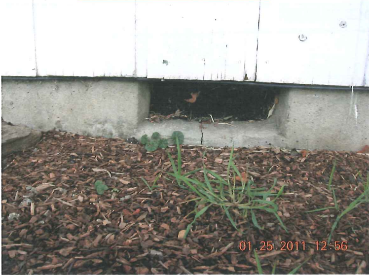
TYPICAL FOUNDATION VENT
