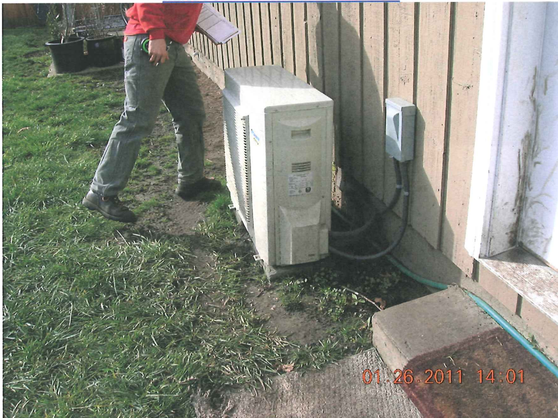
HEAT PUMP ON CONCRETE BLOCKS
