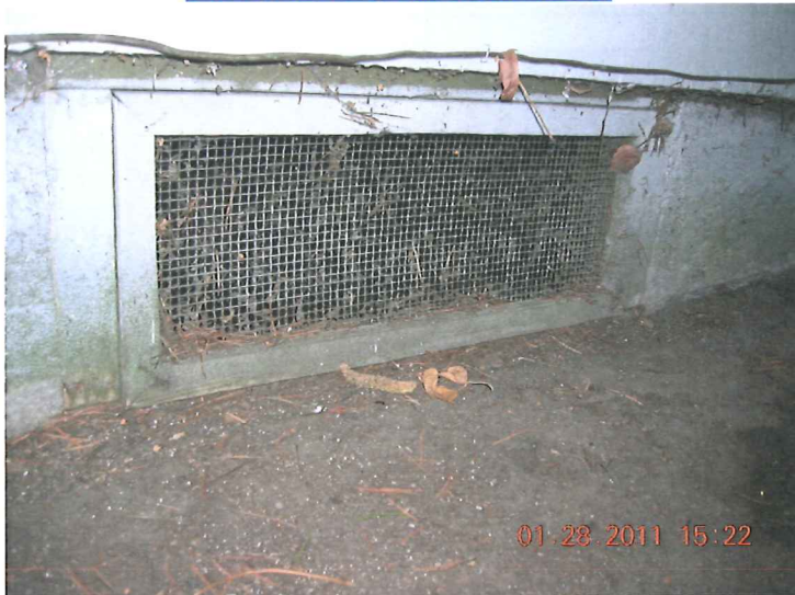
TYPICAL FOUNDATION VENT
