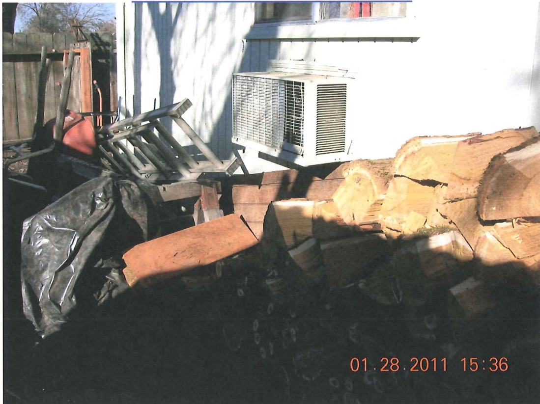
WALL MOUNTED AIR CONDITIONING UNIT
