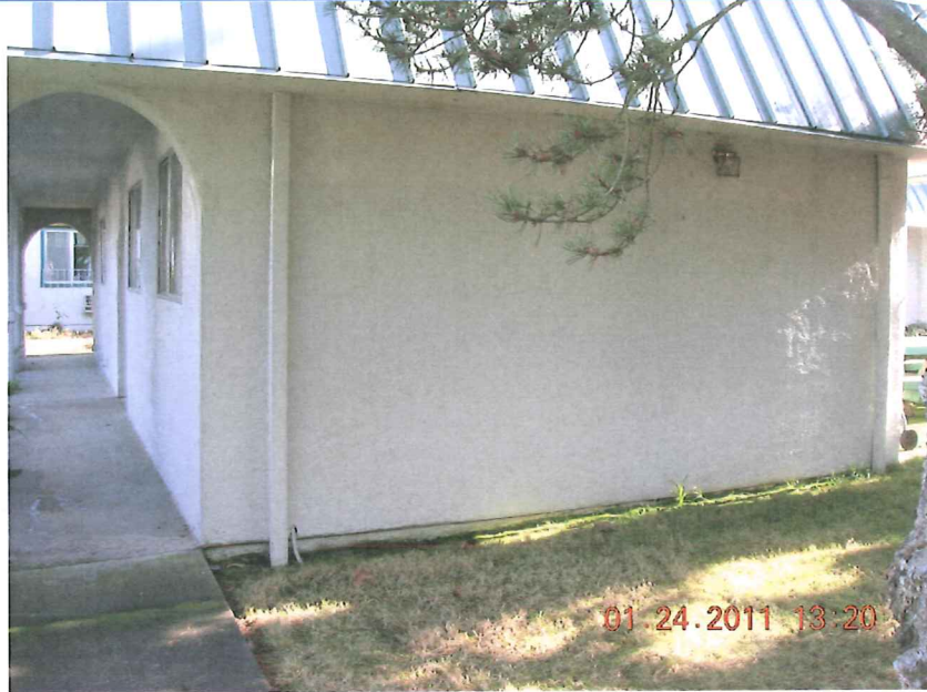
LOOKING WESTERLY AT TOOL ROOM AND COVERED WALKWAY
