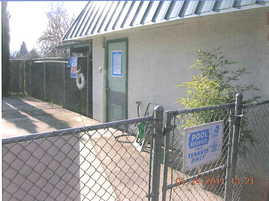
LOOKING SOUTHERLY AT EAST FACE OF POOL ROOM (LOOKING SOUTHERLY)
