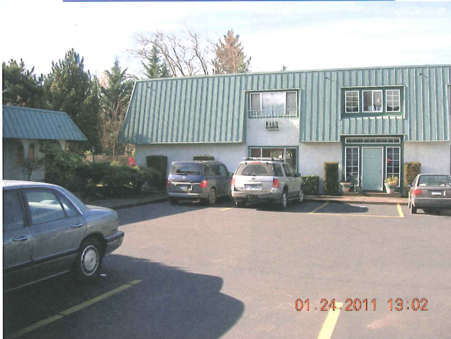
EAST FACE OF BUILDING (SOUTHERLY PORTION)
