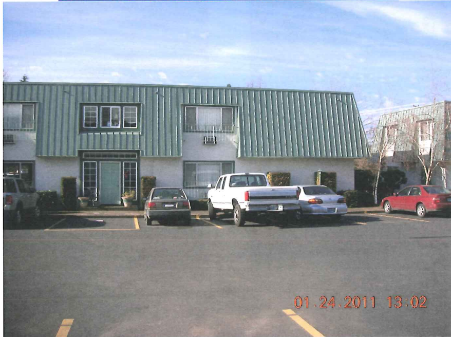
EAST FACE OF BUILDING (NORTHERLY PORTION)
