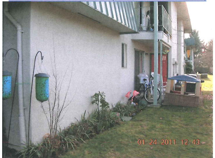
WEST FACE OF BUILDING (LOOKING SOUTHERLY)
