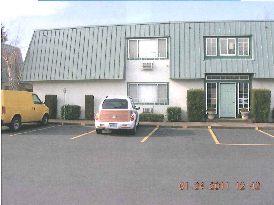
EAST FACE OF BUILDING (SOUTHERLY PORTION)
