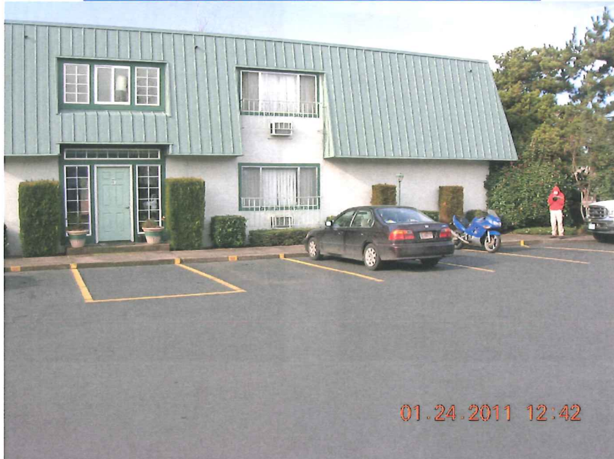
EAST FACE OF BUILDING (NORTHERLY PORTION)
