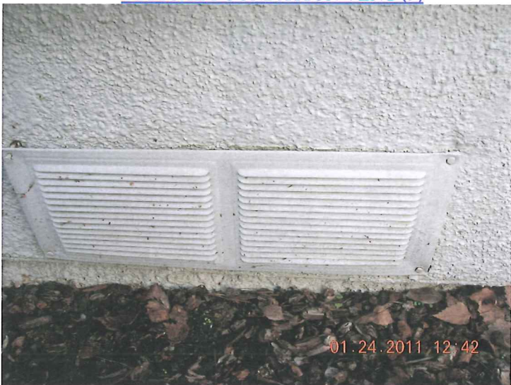
TYPICAL FOUNDATION VENT (9)
