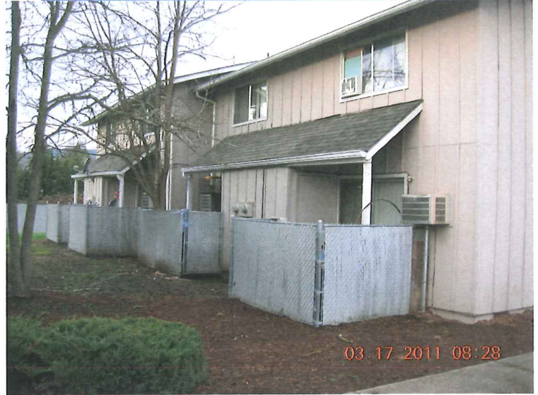
SOUTH FACE OF BUILDING (LOOKING WESTERLY)
