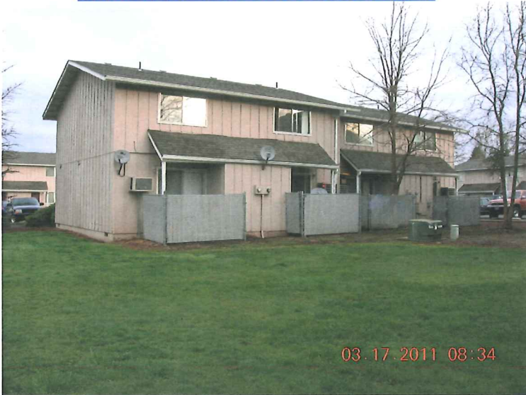
SOUTH AND WEST FACE OF BUILDING
