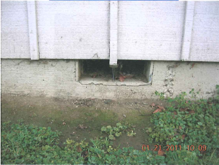
TYPICAL FOUNDATION VENT (9)
