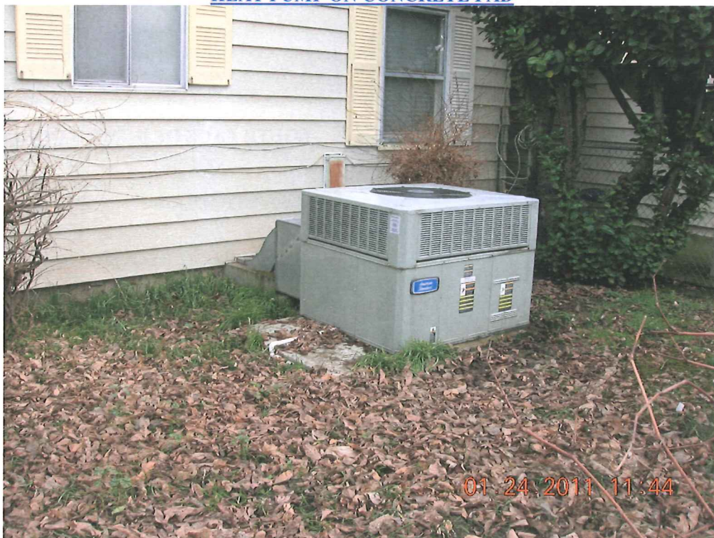
HEAT PUMP ON CONCRETE PAD
