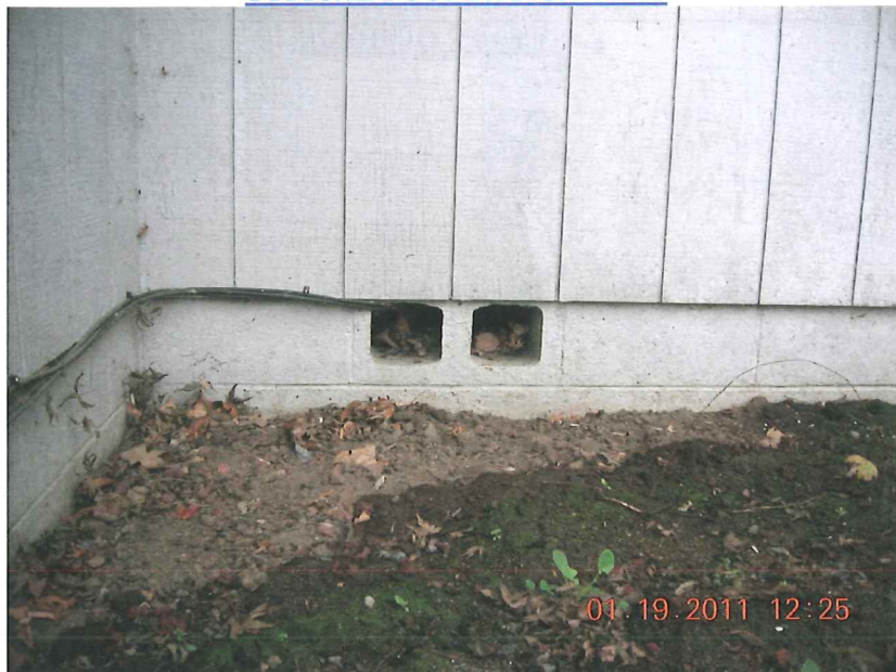
TYPICAL FOUNDATION VENT
