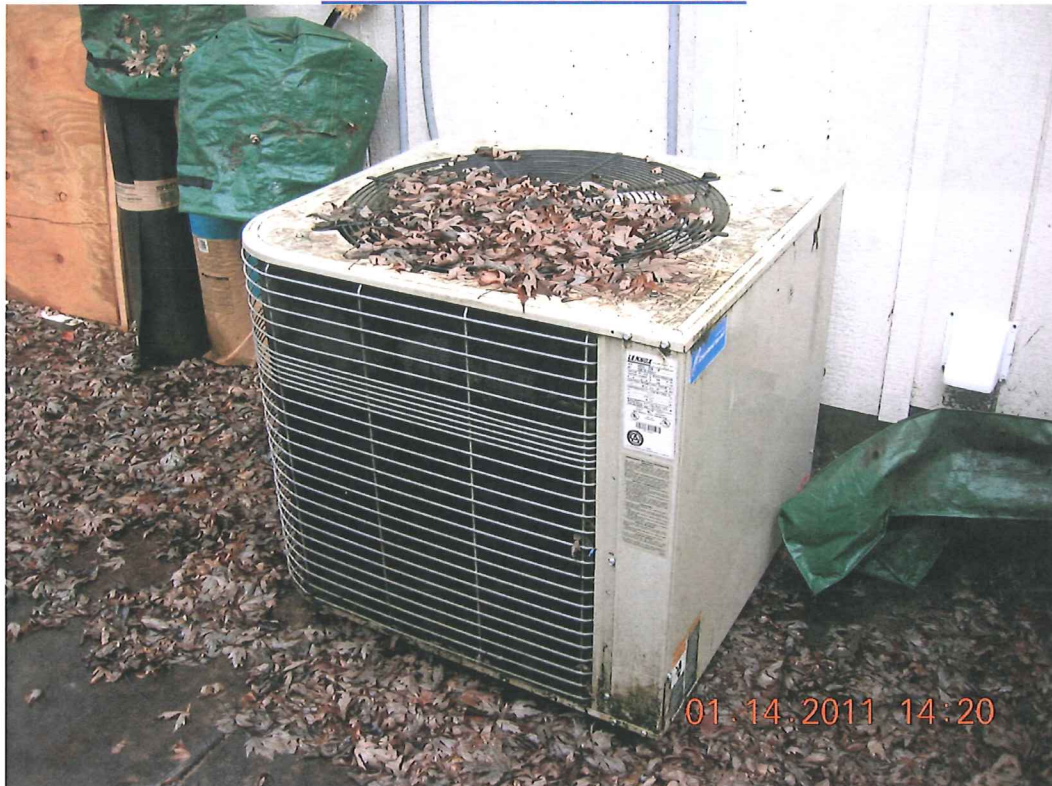
HEAT PUMP ON CONCRETE PAD
