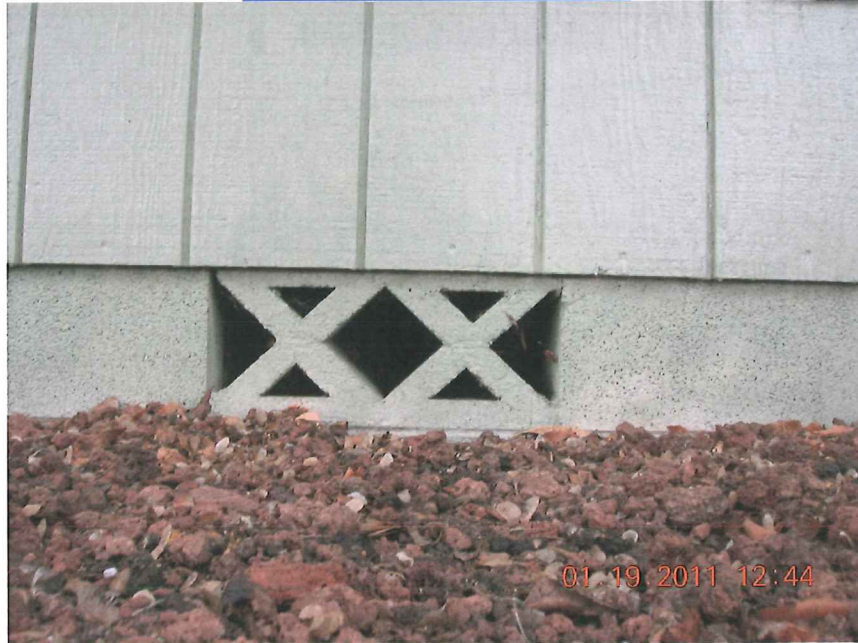
TYPICAL FOUNDATION VENT
