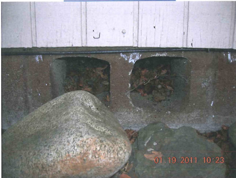
TYPICAL FOUNDATION VENT
