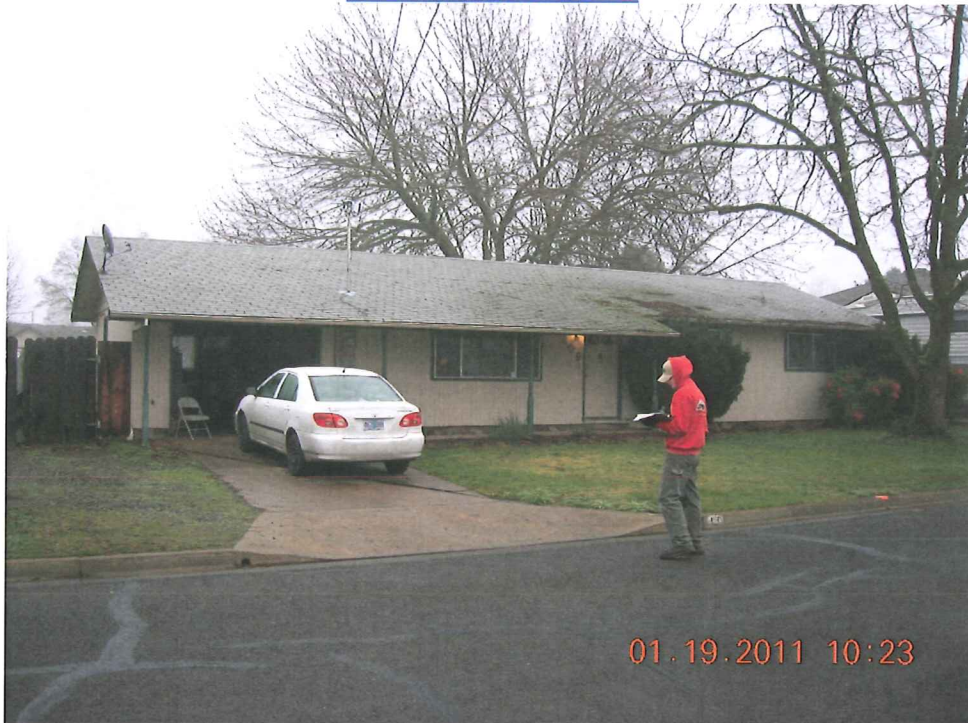
WEST FACE OF HOME
