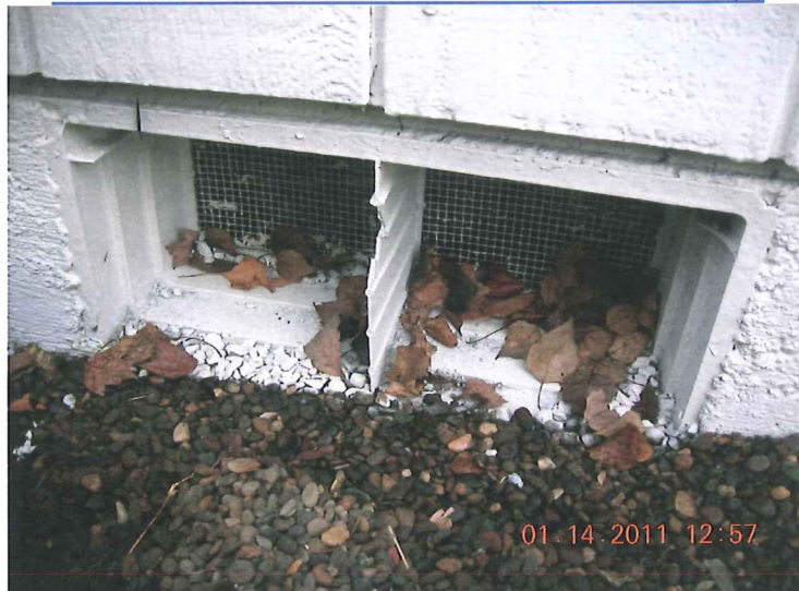
FOUNDATION VENT WITH HARDWARE CLOTH (4)
