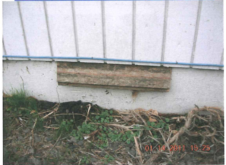
FOUNDATION VENT COVERED WITH A BOARD (9)
