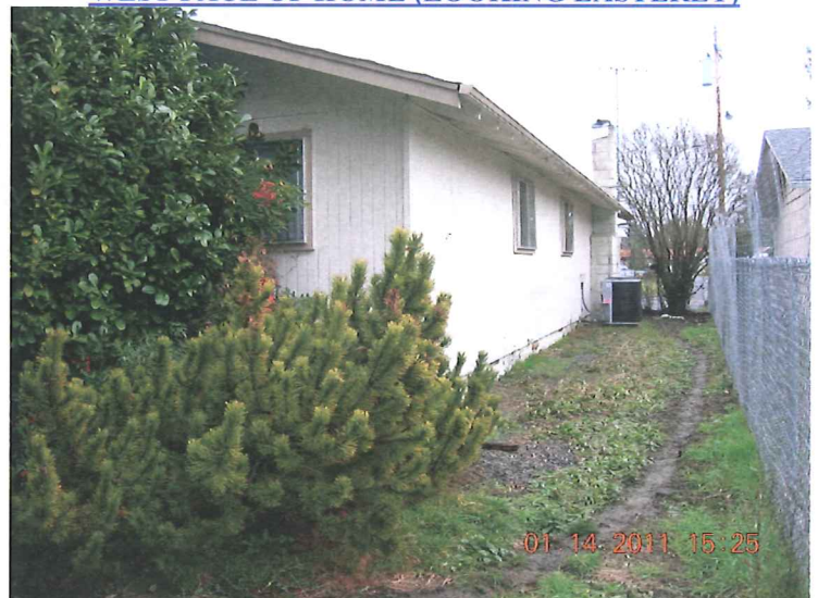
WEST FACE OF HOME (LOOKING EASTERLY)
