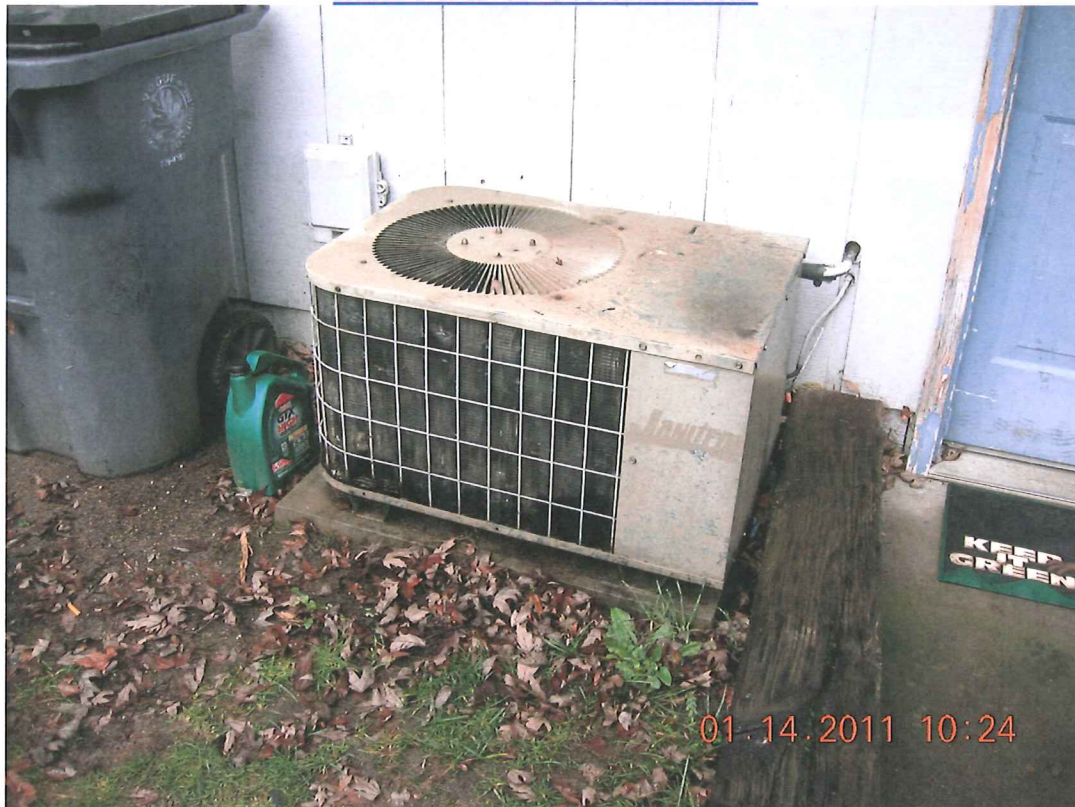
HEAT PUMP ON CONCRETE PAD
