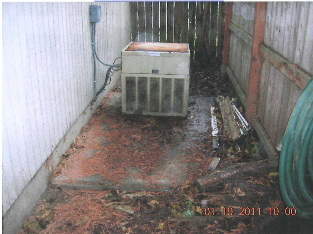
HEAT PUMP ON CONCRETE PAD
