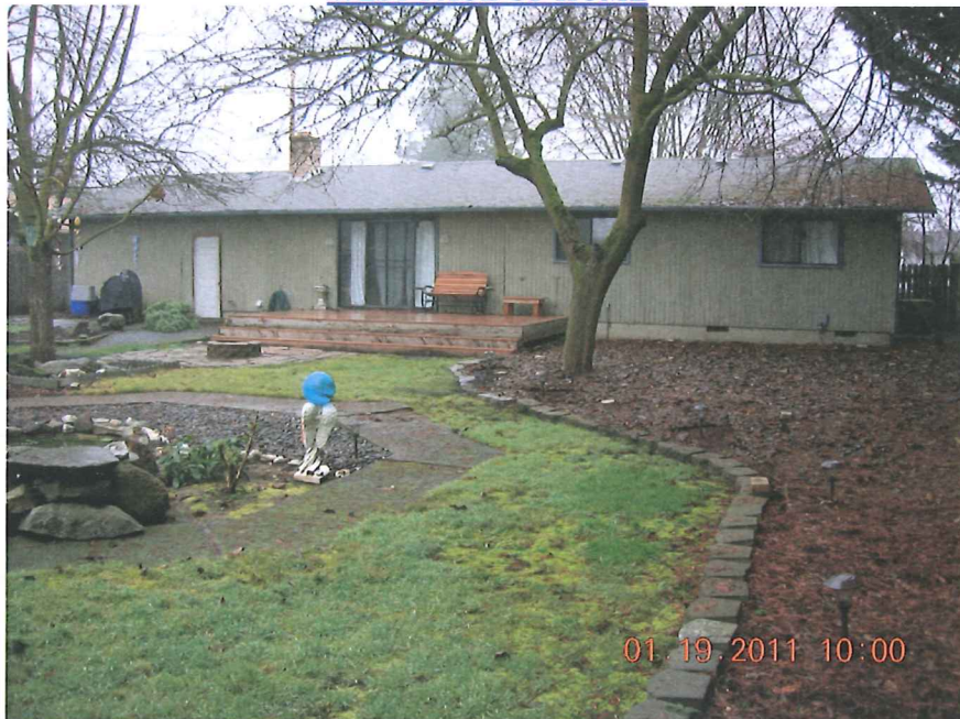
WEST FACE OF HOME
