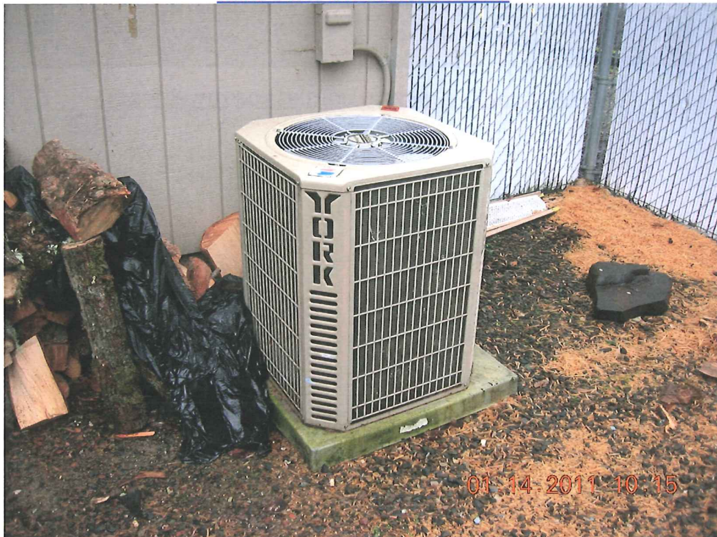
HEAT PUMP ON CONCRETE PAD
