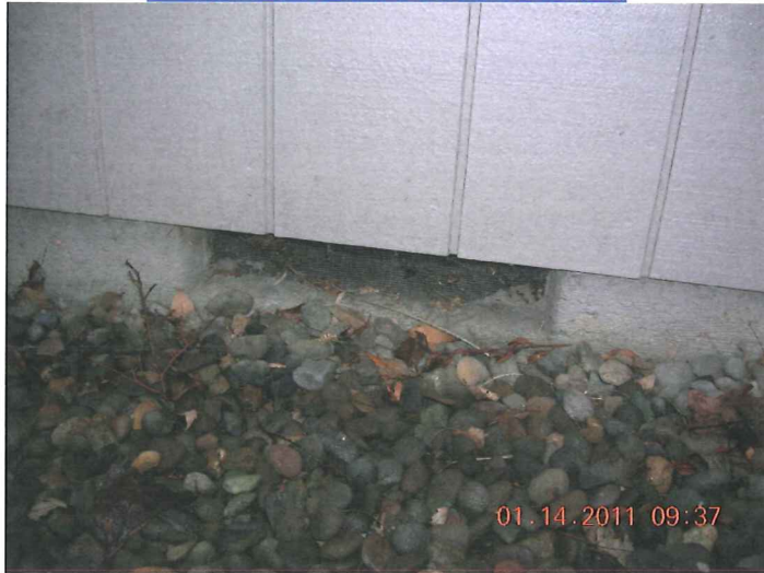
TYPICAL FOUNDATION VENT (11)
