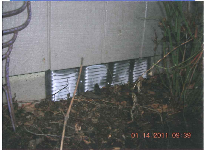
FOUNDATION VENT WITH LOUVERED COVER (2)
