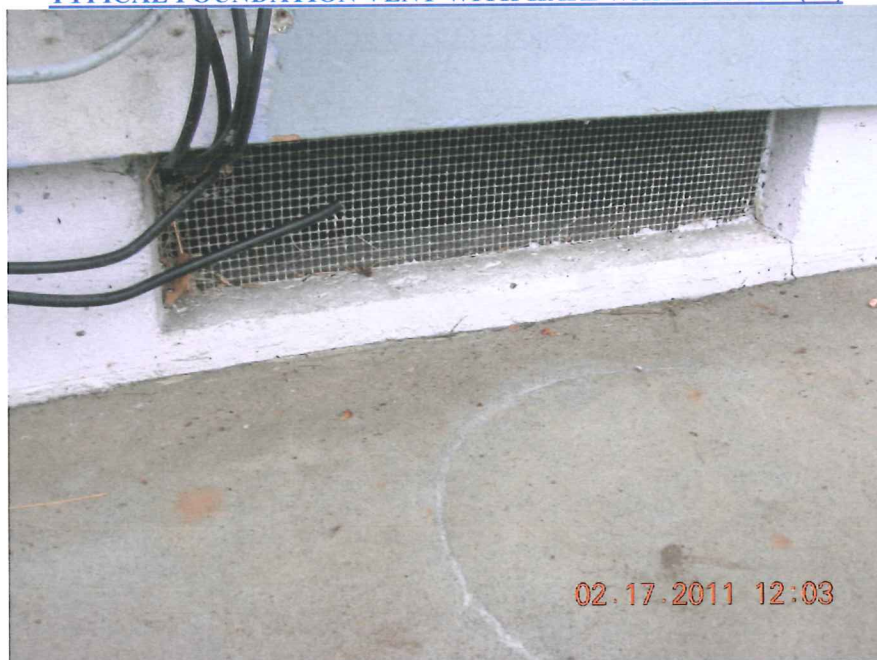
TYPICAL FOUNDATION VENT WITH HARDWARE CLOTH (11)
