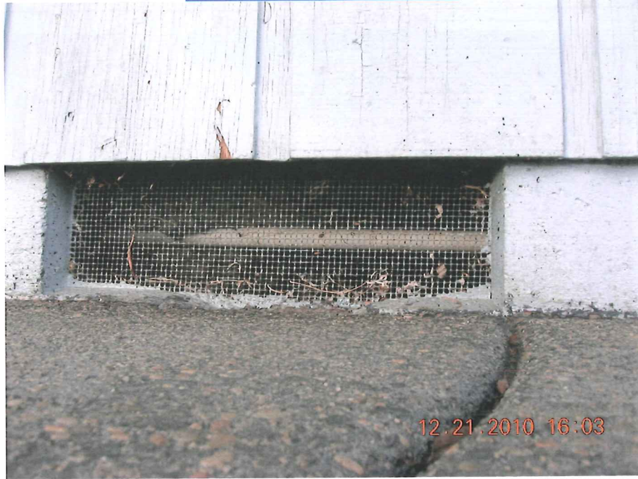
TYPICAL FOUNDATION VENT
