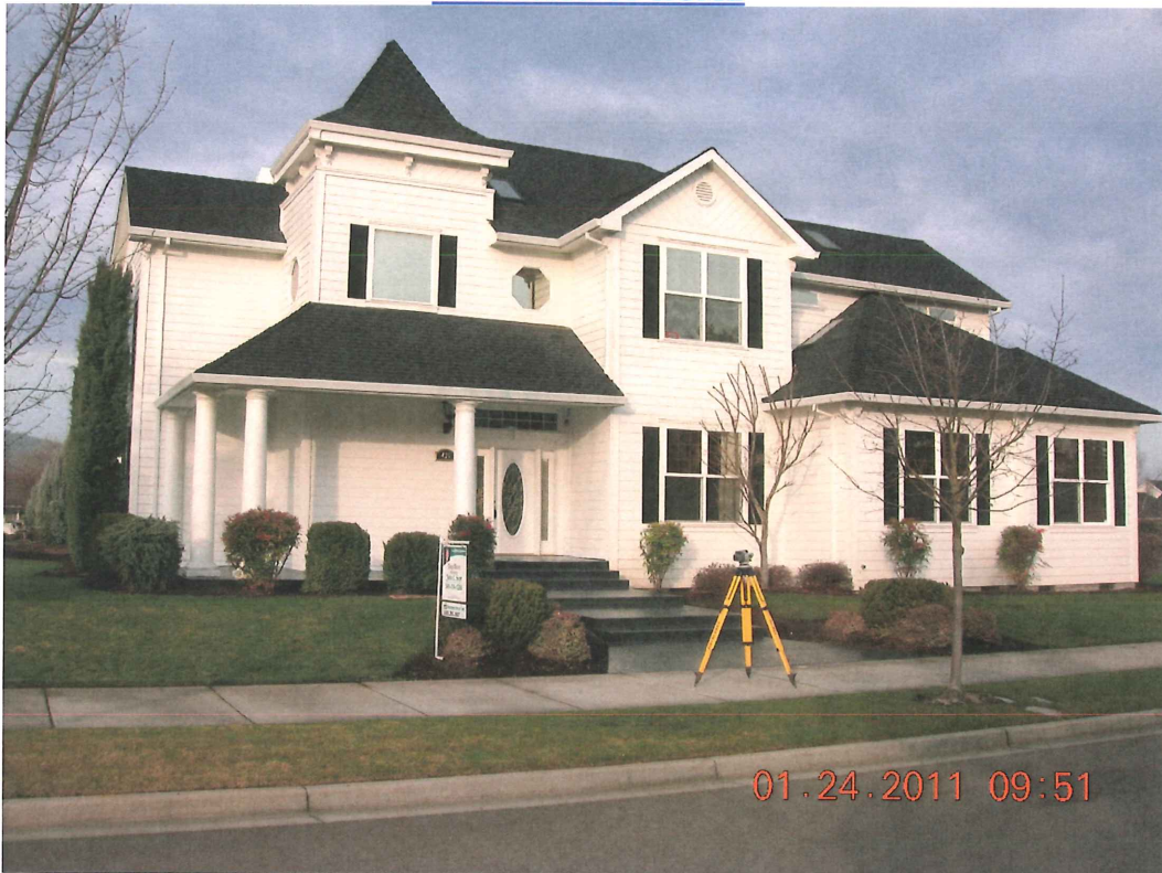
EAST FACE OF HOME
