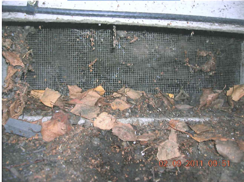
TYPICAL FOUNDATION VENT
