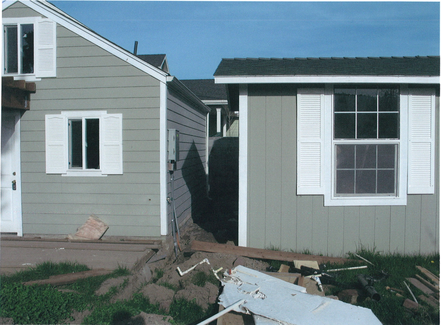
Southwest side of apartment next to shed. Underground power connection. Jackson Creek is to the south (right). Date taken March 30, 2007.
