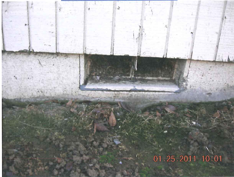
TYPICAL FOUNDATION VENT
