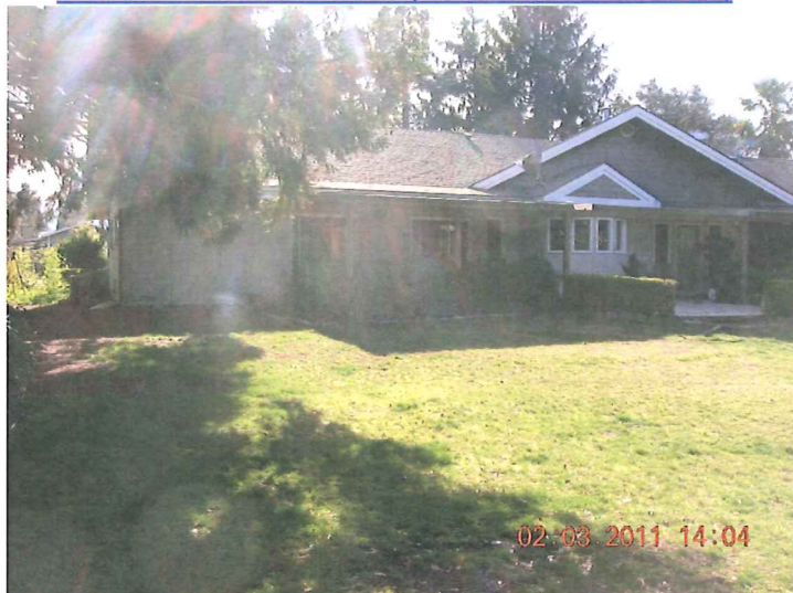
NORTH FACE OF HOME (EASTERLY PORTION)
