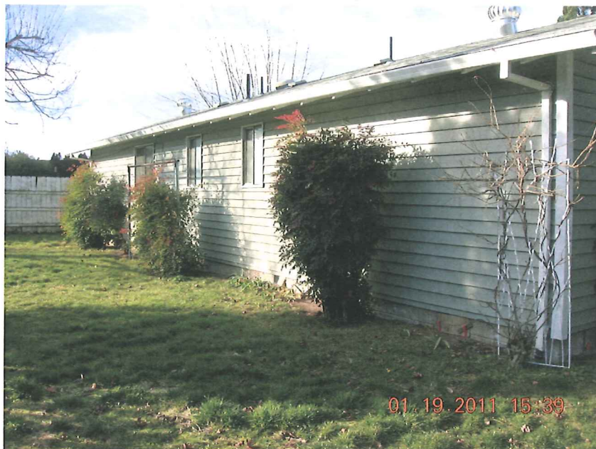
SOUTH FACE OF HOME (LOOKING WESTERLY)
