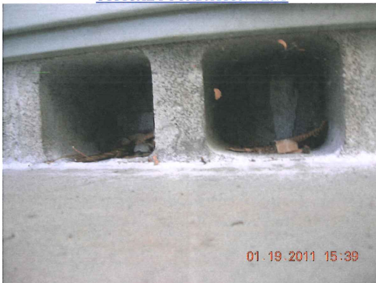
TYPICAL FOUNDATION VENT
