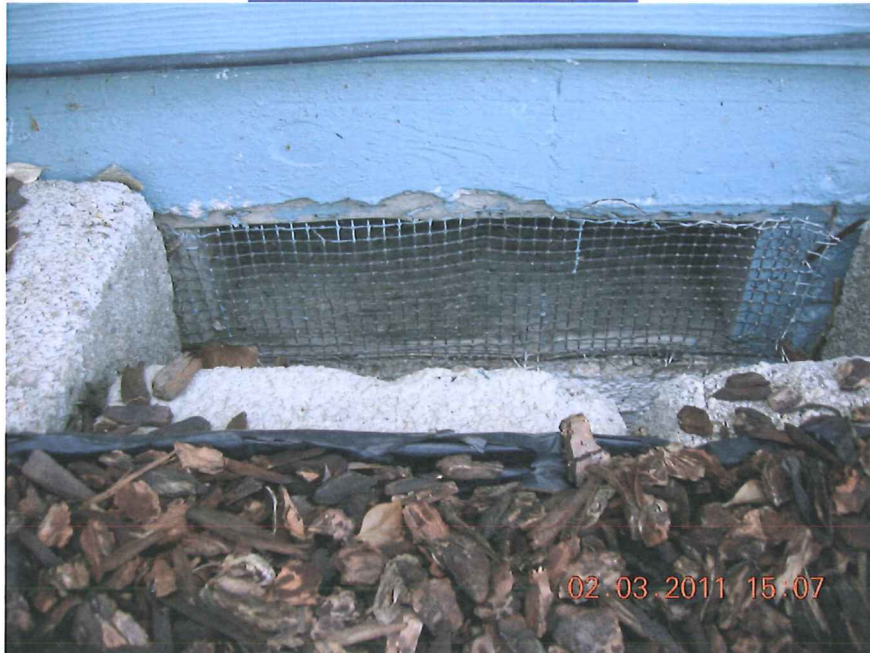
TYPICAL FOUNDATION VENT
