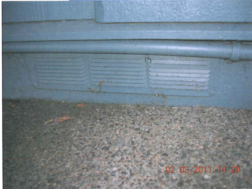
TYPICAL FOUNDATION VENT
