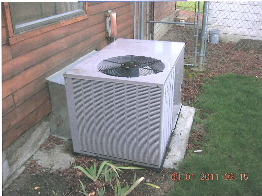
HEAT PUMP ON CONCRETE PAD
