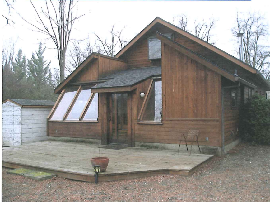
SOUTH FACE OF HOME (LOOKING NORTH WESTERLY)
