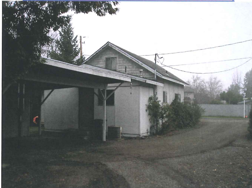
SOUTH FACE OF HOME (LOOKING NORTH WESTERLY)
