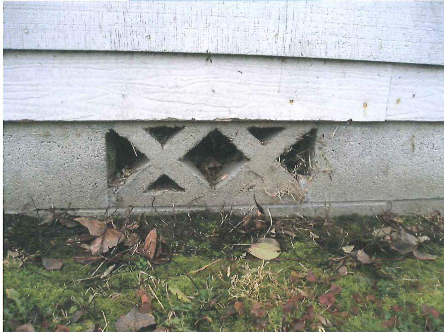
TYPICAL FOUNDATION VENT
