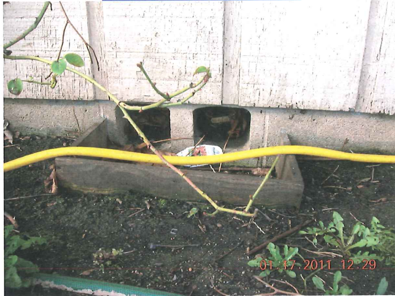
TYPICAL FOUNDATION VENT
