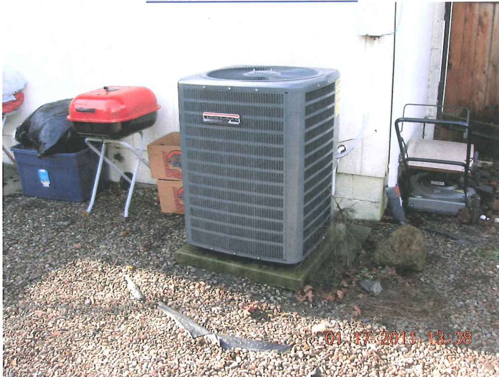
HEAT PUMP ON CONCRETE PAD
